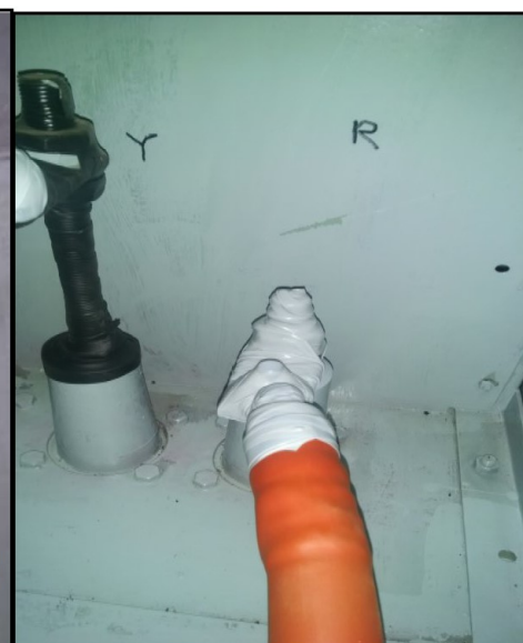
(Application of Silicon)
