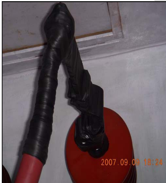
Application of EPR tape (3M-Scotch-130C)
