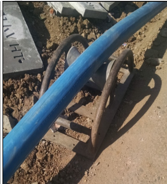
(Rollers for cable pulling)
