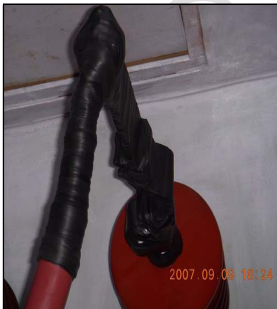
Application of EPR tape (3M-Scotch-130C)
