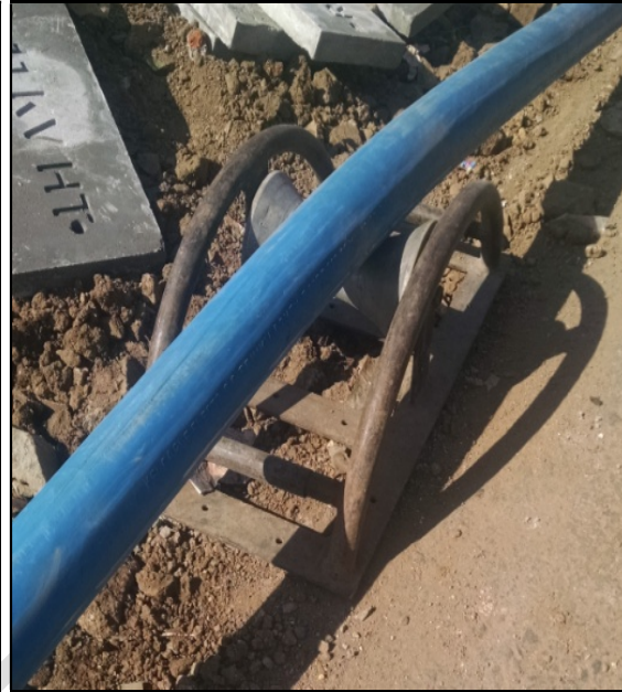
(Rollers for cable pulling)
