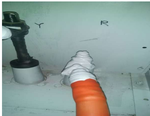
Application of Silicon tape
