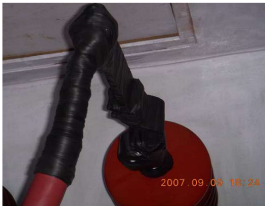
Application of EPR tape (3M-Scotch-130C)
