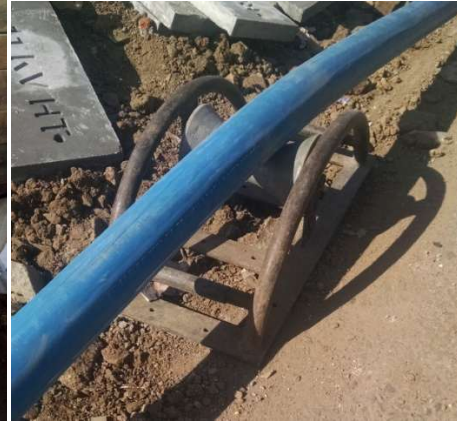
(Rollers for cable pulling)
